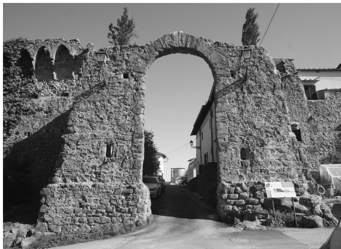
Figure 12. (above) Malmantile, Porta Pisana with the stretch of walls where the corbels are still present and part of the walkway.
