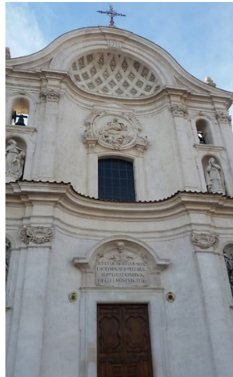
Fig.5. Church of S. Maria del Suffragio, Aquila, Italy, Façade restoration with work completed. [12]
