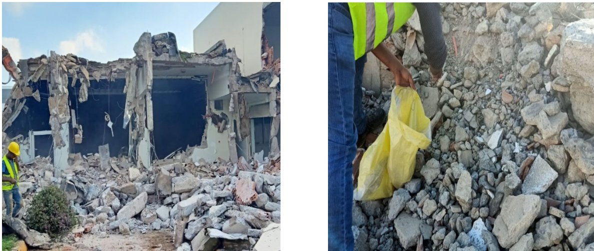
Fig. 1. The collection of CDWs from a demolition site in Casablanca.
